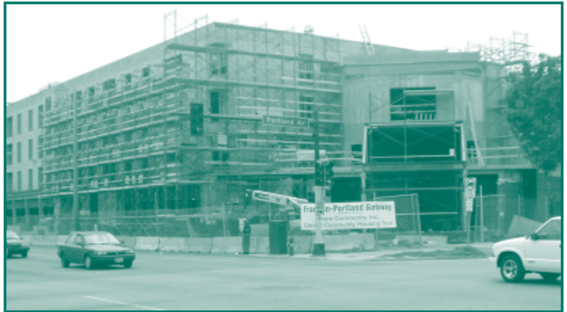
Children's Village Center under construction at Franklin and Portland Avenues.
